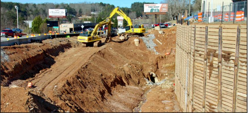
GDOT is planning to spend \$5.1 million to install a new stormwater pipe after the old one burst in a rainstorm last August, contributing to a massive sinkhole at Murphy Highway and GA 515. Photo by Shawn Jarrard
